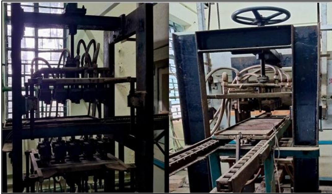
Fig.3.1.3 Nozzle Bank and Cooling Bay
