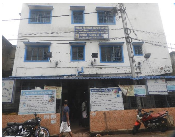
Plate 5.m: Nearest Health center for Narkel Danga Canal East and West Road (Along the Canal Line, Registered and Unregistered Slum)
