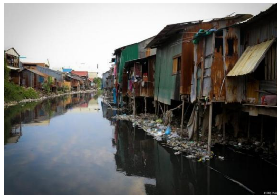
Plate 5.z: Sewerage Condition of Narkel Danga Canal West Road (Along the Canal Line, Unregistered Slum)
