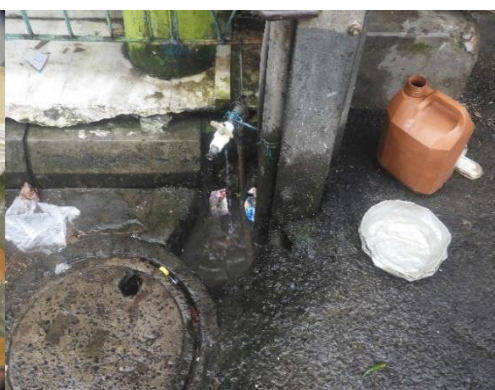
Plate 5.d: Madhobtala Lane Bustee (Along the Railway Line, Unregistered Slum)
