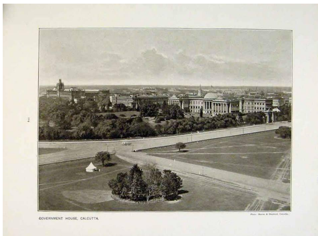
Fig 1.2: A panoramic view of Calcutta from the Ochterlony Monument, with the Governor House, Town Hall and Supreme Court in prominent view. 1890s.
