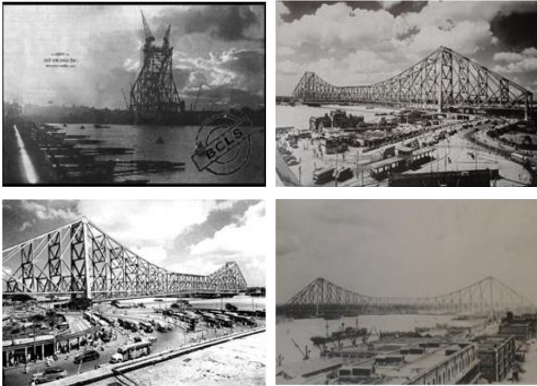
Fig 4.13: Clockwise from Top Left A photograph of ‘Howrah Bridge under Construction’, says the embedded caption, 1942; The bridge from Strand Road by Jayant Patel, 1948; The ‘new’ Howrah Bridge by Gurney Nyss, 1946; Howrah bridge from station side, Ahmed Ali, 1959.
