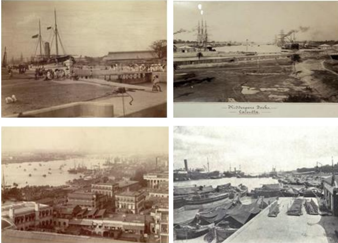
Fig 4.8: Above left and right Kidderpore dock in a state of construction in its very early days, from private album, 1890s; Below right and left The Outram Jetty on the strand with anchored small boats to ferry stuff from the warehouses, P Bose & Company; Hooghly from Supreme Court, looking north over the rooftops of export and import jetties; Johnston and Hoffman.
