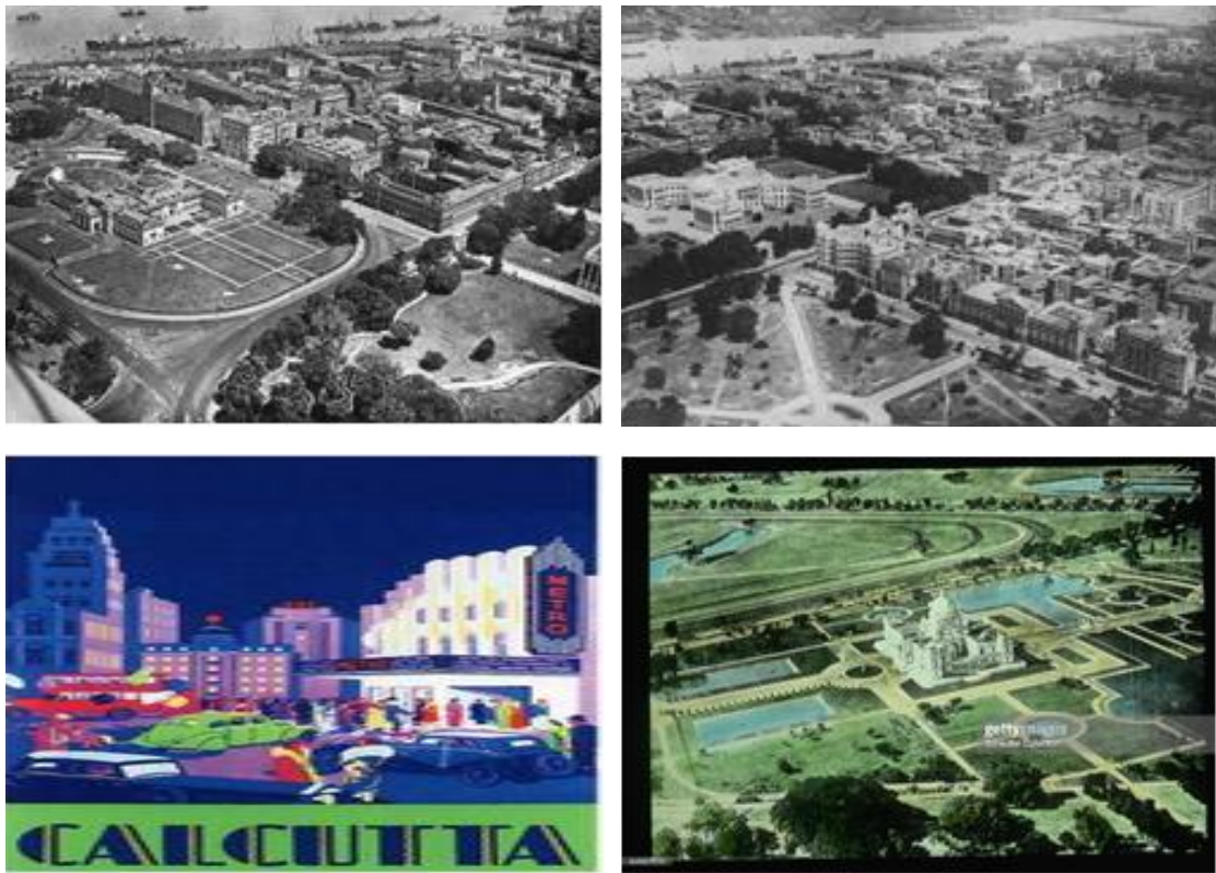
Fig 5.11: Clockwise from top left Grand buildings on the banks of the Hooghly River in Calcutta circa 1930; An aerial view of Calcutta, showing Government House (large white structure to the left), the Post Office (with white dome) and the Esplanade Curzon Gardens in the foreground, 1932; Aerial view of the Palace and of Queen Victoria and surrounding grounds, Calcutta 1932-1937; A travel poster of Calcutta, 1938, highlighting the art-deco distinctions (Tower house, GEC House, Victoria House and Metro Cinema ) of its downtown. The aerial views courtesy Getty Images; the poster from Library of Congress.
