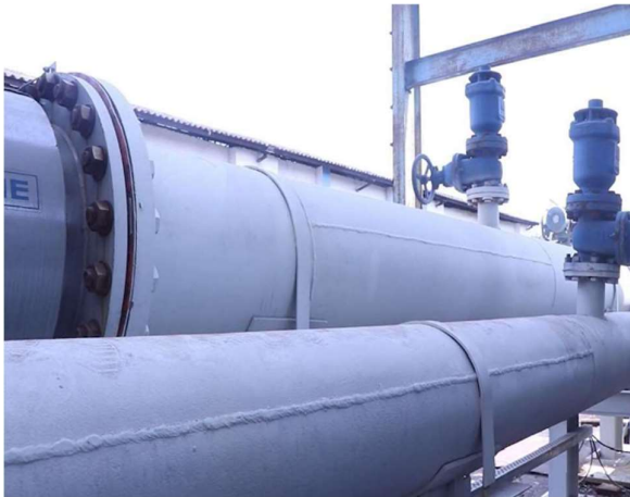
TEST PIPE LINE
