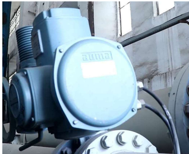
REGULATION VALVE ACTUATOR
